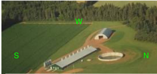
Figure 1: Pig Production Innovation Group Swine Facility - Union Road PEI.
